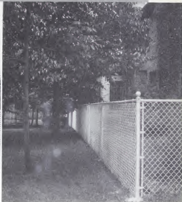
See how this long division fence definitely and pleasingly marks off the limits of the property. The tubular steel corner post is set firmly in concrete and it will not give in any direction. The other posts are in concrete too.
